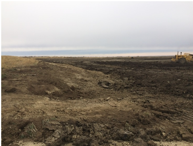
Photo 2: 2017 Columbus Phase 16 AML Project – Site 1. Facing west, shows a scraper levelling topsoil where the former pit meets active farmland.
